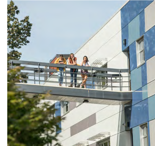
Lansdowne Campus - Overhead Link
